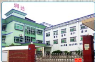
厂区一角 A Corner of Factory
