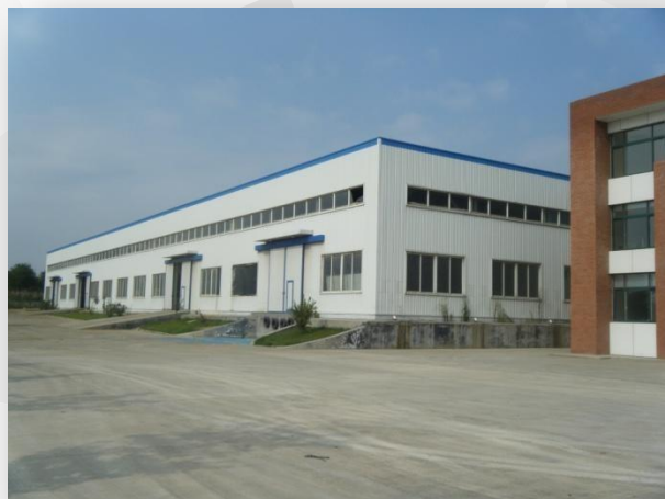
Phase one plant
